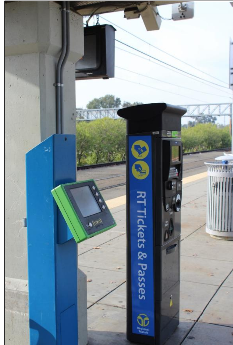
Ticketing machines are located far from the stairs and elevators, causing missed transfers.
