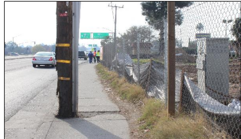
Broken concrete and utility poles on the sidewalk are barriers for pedestrians with mobility disabilities.
