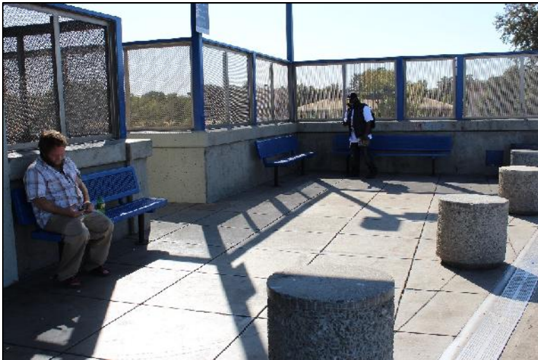
Seating areas are unshaded and exposed to the elements.
