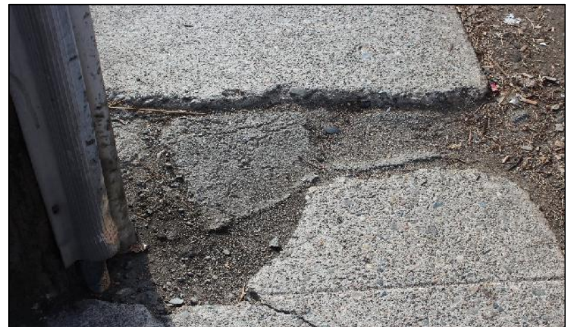
Repaving sidewalks and asphalt are priorities for ADA access.
